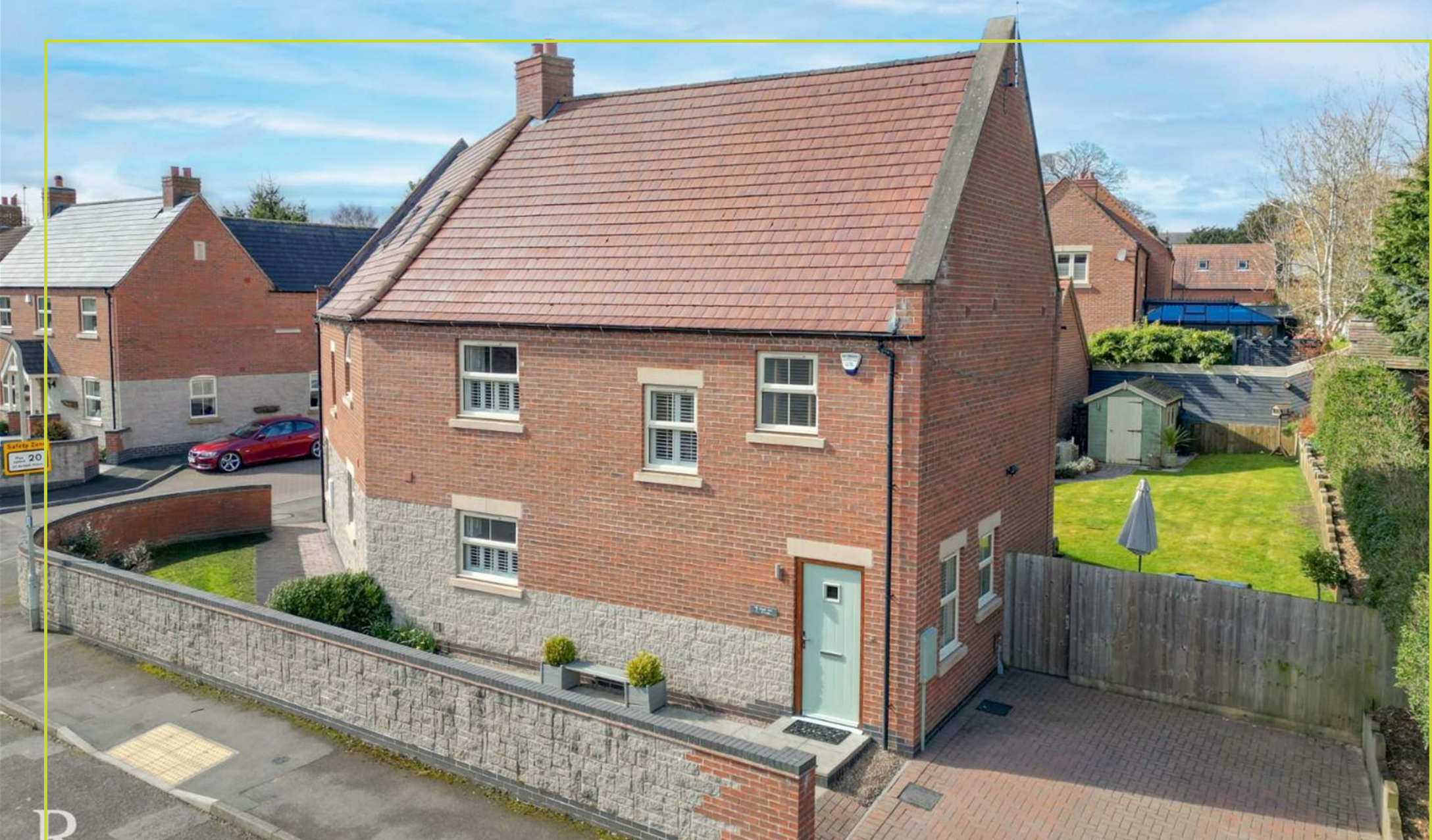
Cloud View Cottage, 7 Manor Drive | LE65 1RN | Offers In The Region Of £320,000
