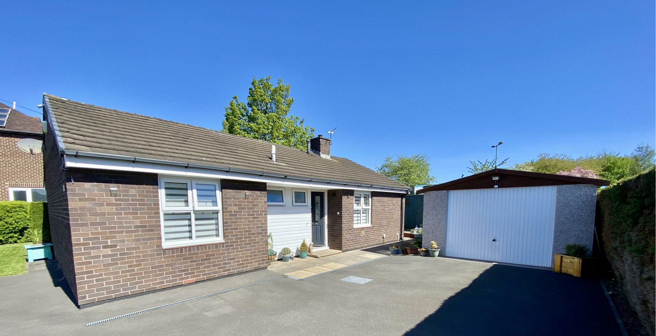
School Bungalow Wellhouse Lane, Mirfield, WF14 0BE Asking Price £325,000
