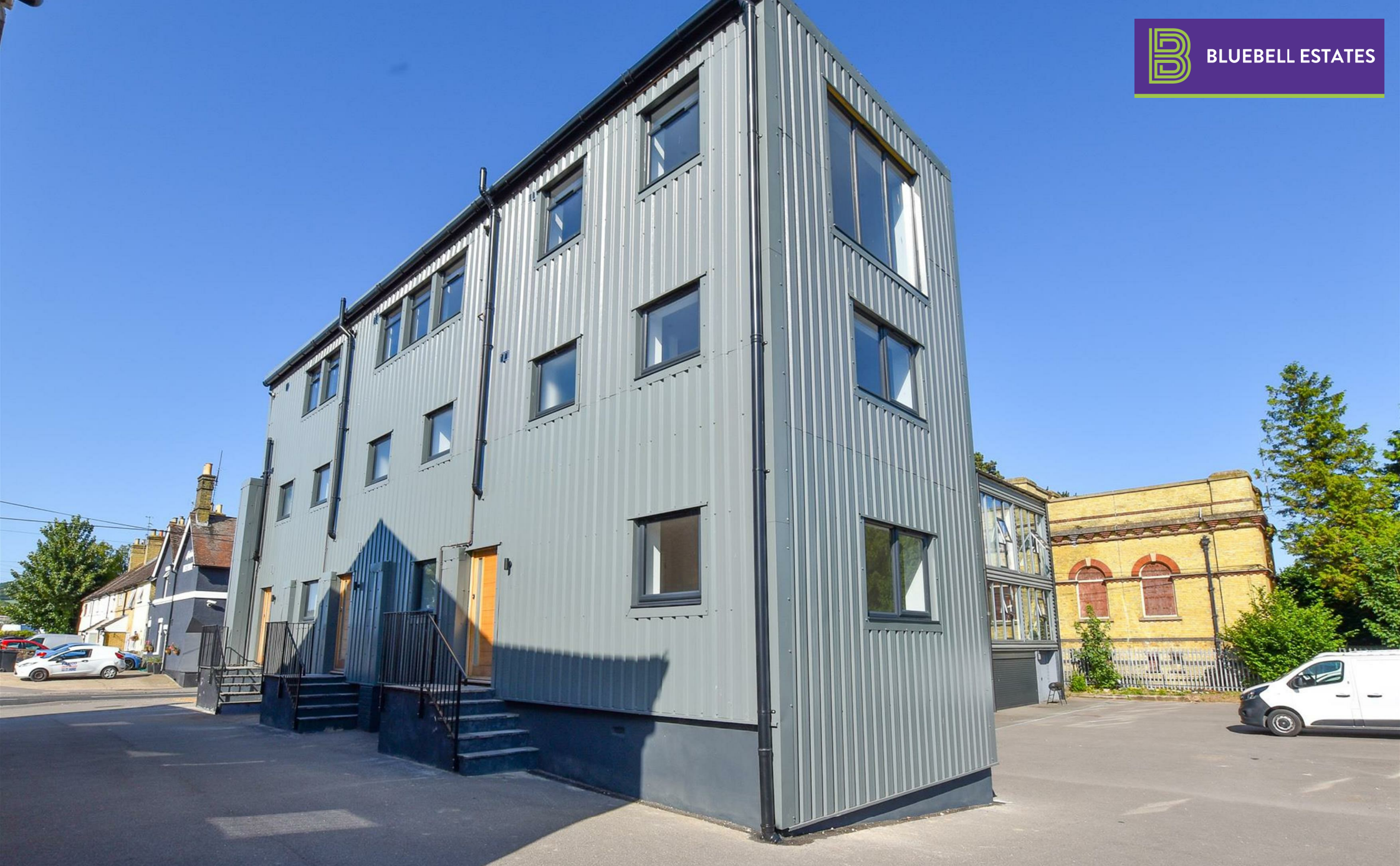
The Pump House, Forstal Road, Aylesford, ME20 7AH £260,000
