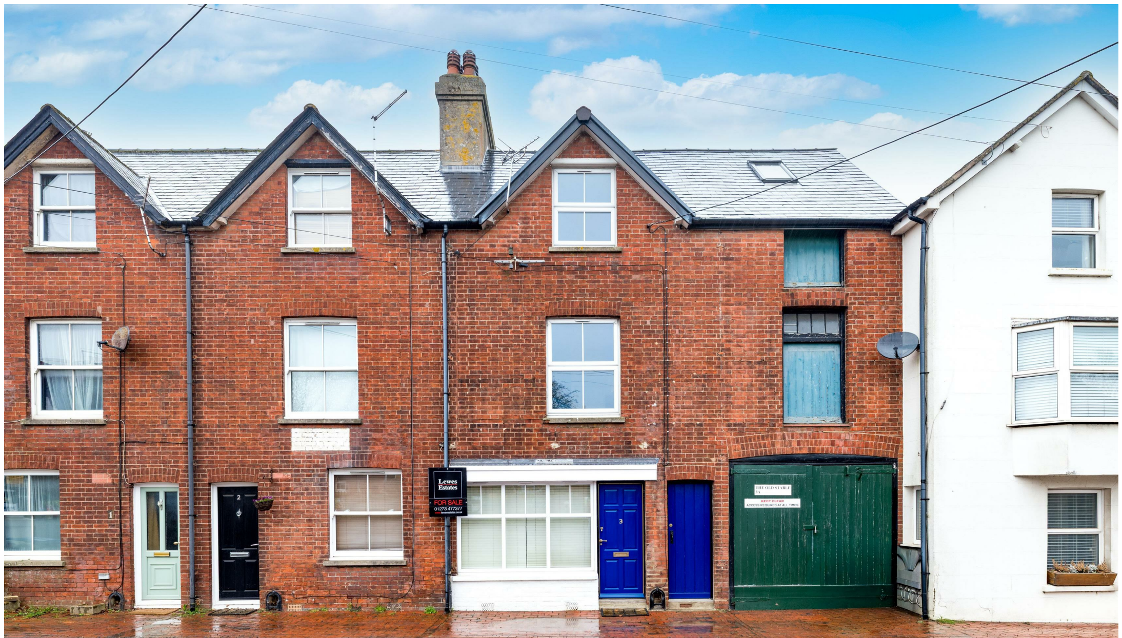
Wellington Cottages, Cooksbridge
